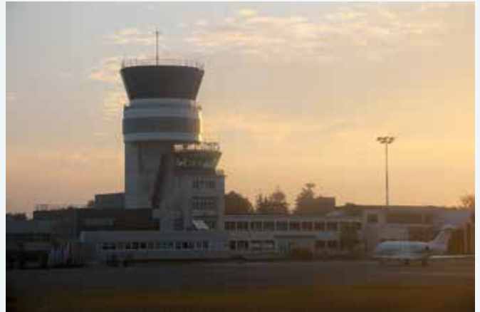
Pau-Pyrénées control tower in the early hours of the morning.
