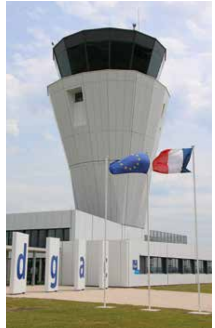
Beauvais-Tillé airport control tower operational since 22 January 2019.
