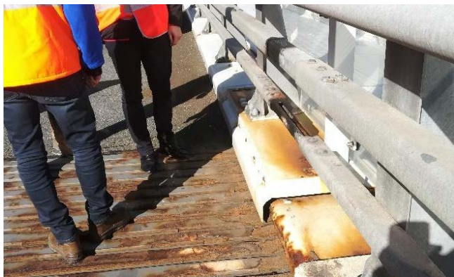
Joint de dilatation sud, A75 sens 2 PR 222+400 Millau (12), 26/10/2020, B. Velty
