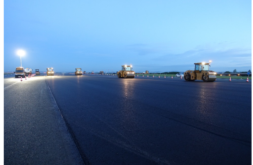
RWY 09L/27R - Reconstruction of the surface course
