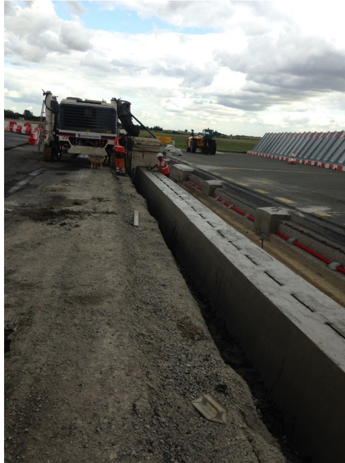
TAXIWAY ROMEO – Reconstruction of deicing pad gutters
