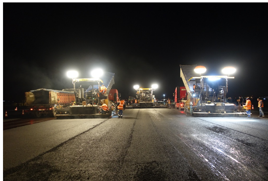
RWY 09L/27R - Reconstruction of the surface course
