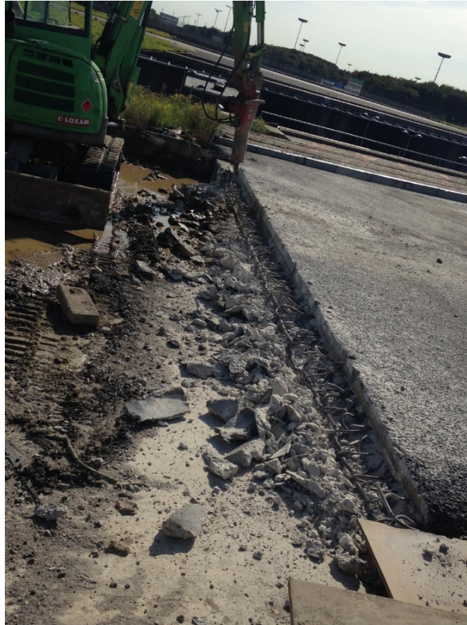
TAXIWAY BRAVO – Complete reconstruction
