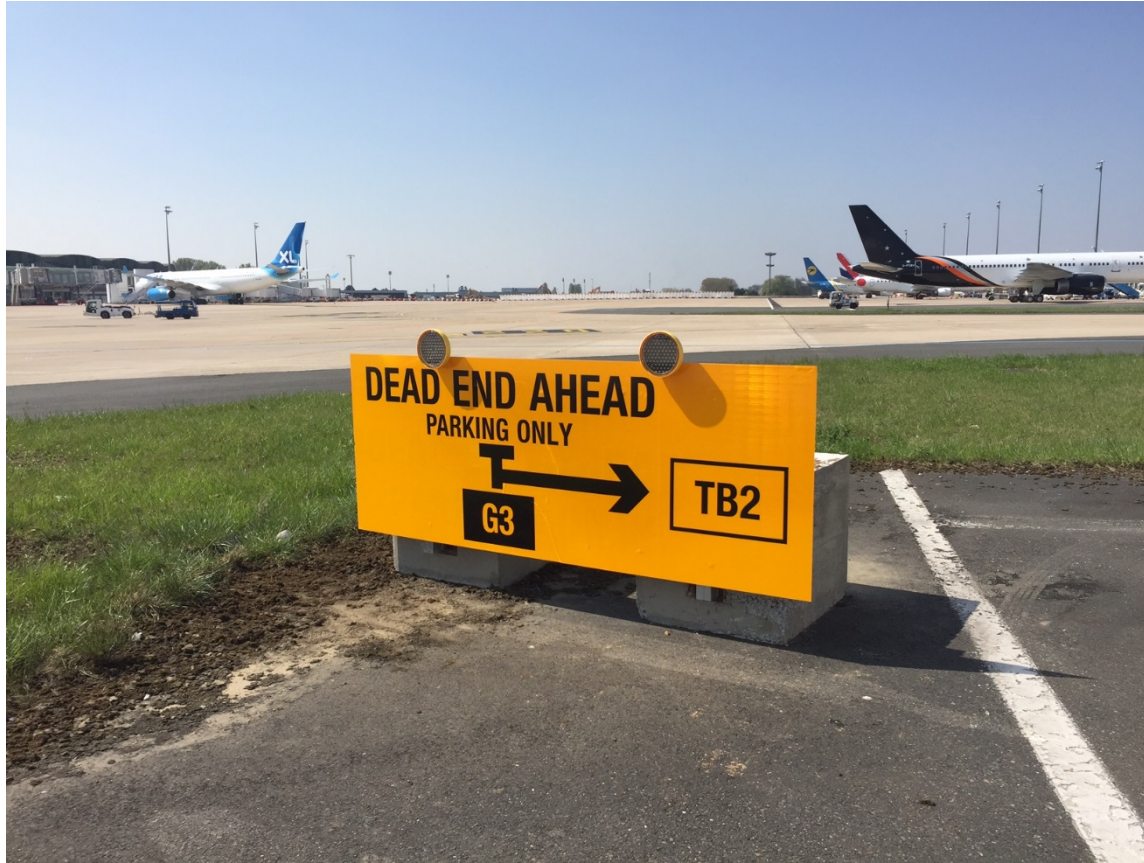
TAXIWAY G3 – Complete rehabilitation
