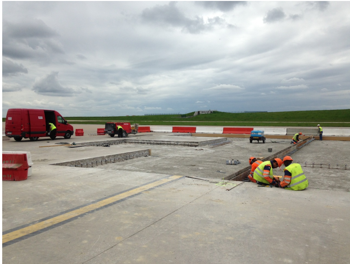
TAXIWAY QUEBEC – Refurbishment of concrete slabs
