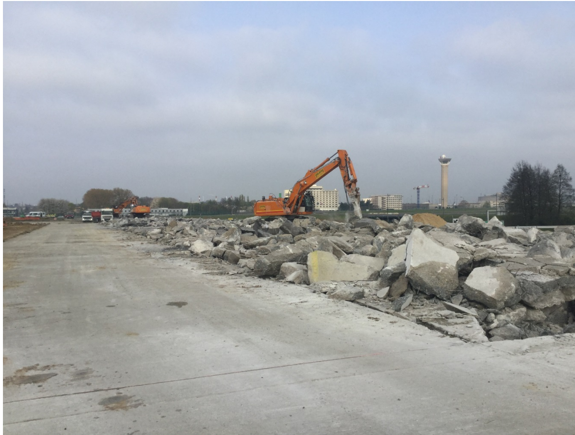
TAXIWAY G3 – Complete rehabilitation
