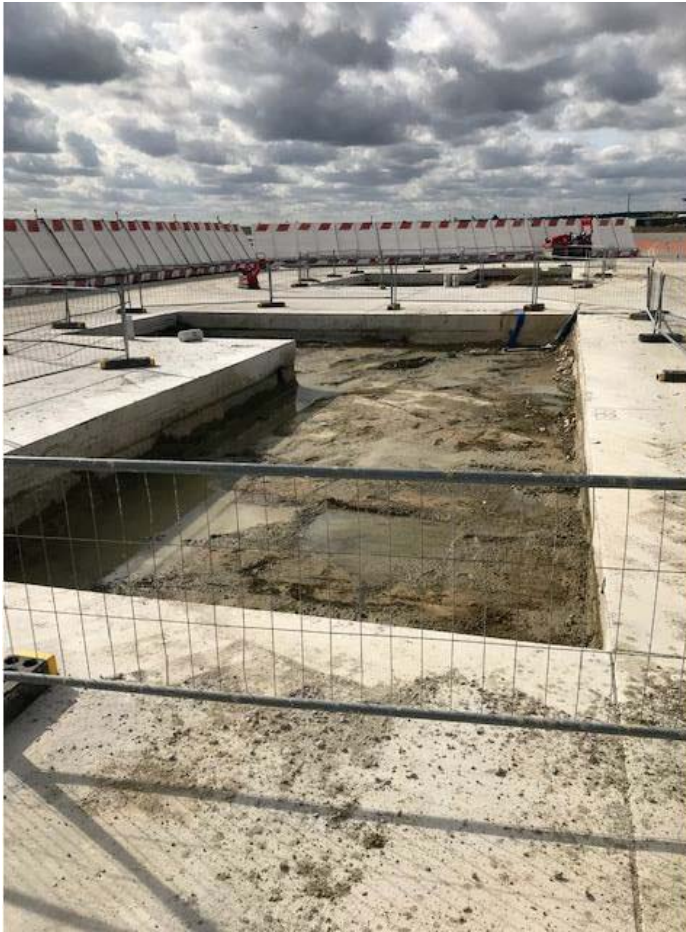
TAXIWAY ROMEO :19 concrete slabs - 3 weeks
