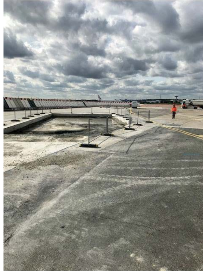
TAXIWAY ROMEO :19 concrete slabs - 3 weeks
