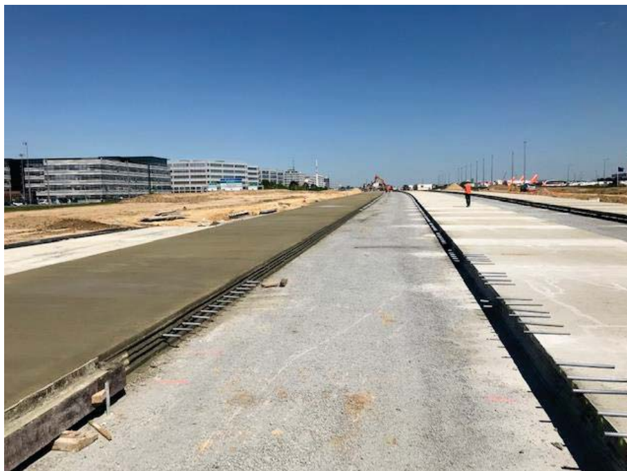
TAXIWAY ECHO: complete rehabilitation of concrete surface and lights on 7000 m 2
